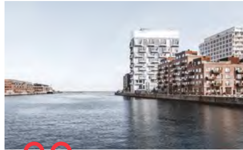
82 Silo in Copenhagen Microtopping®
